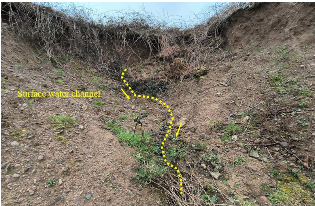
Figure 6 Surface water channel in a landslide scarp
