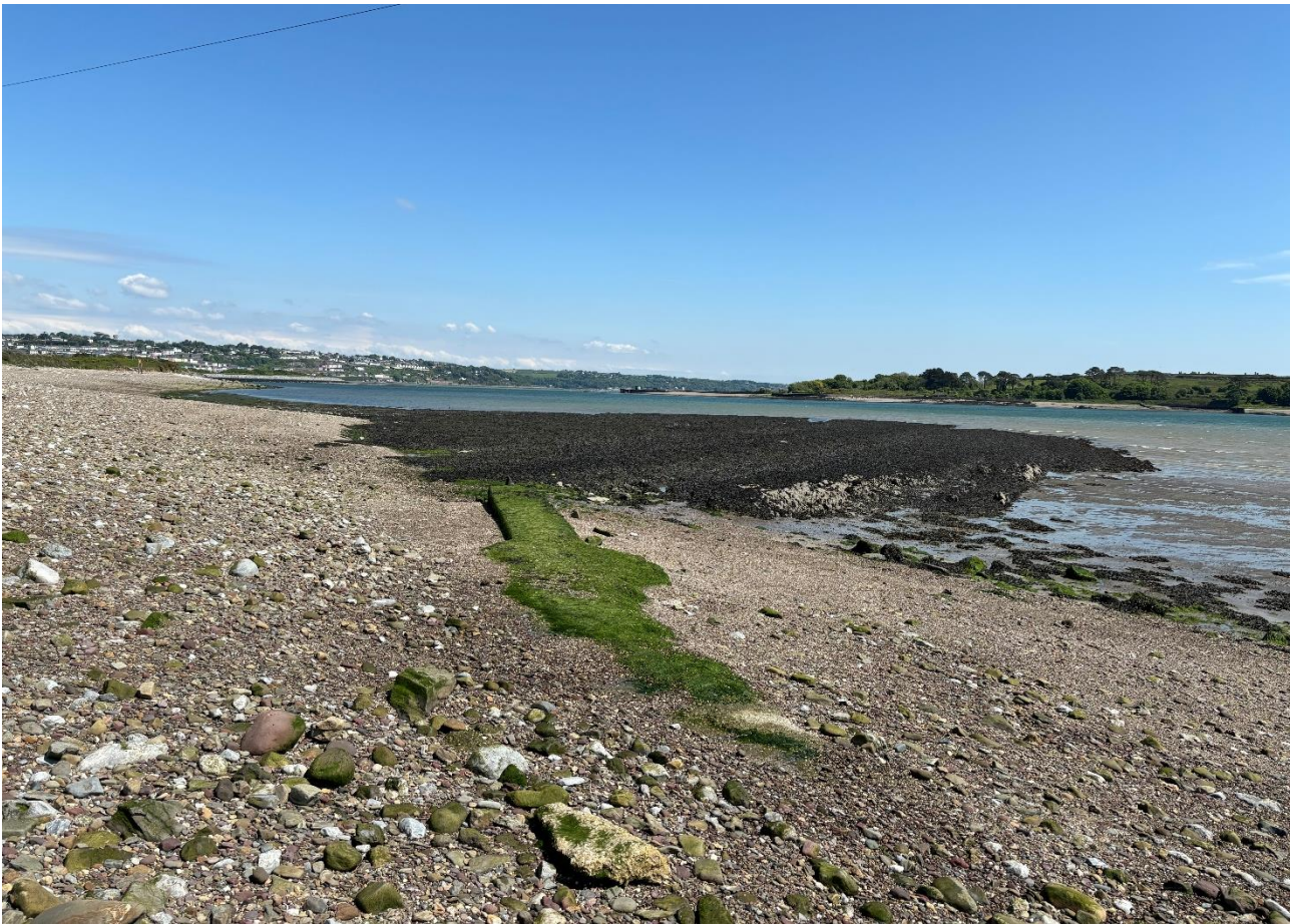
Figure 34 Drainage network outfall
