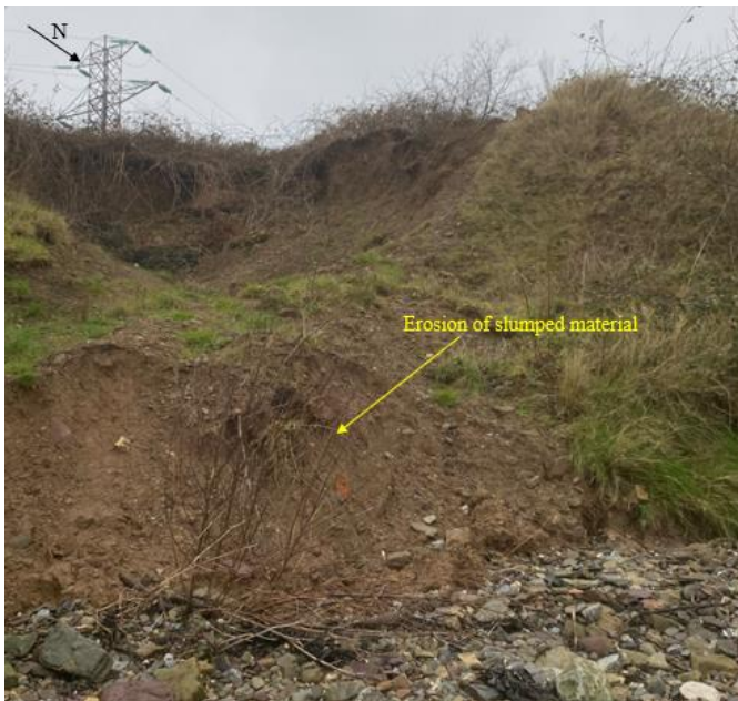
Figure 7 Landslide between Section F and G
