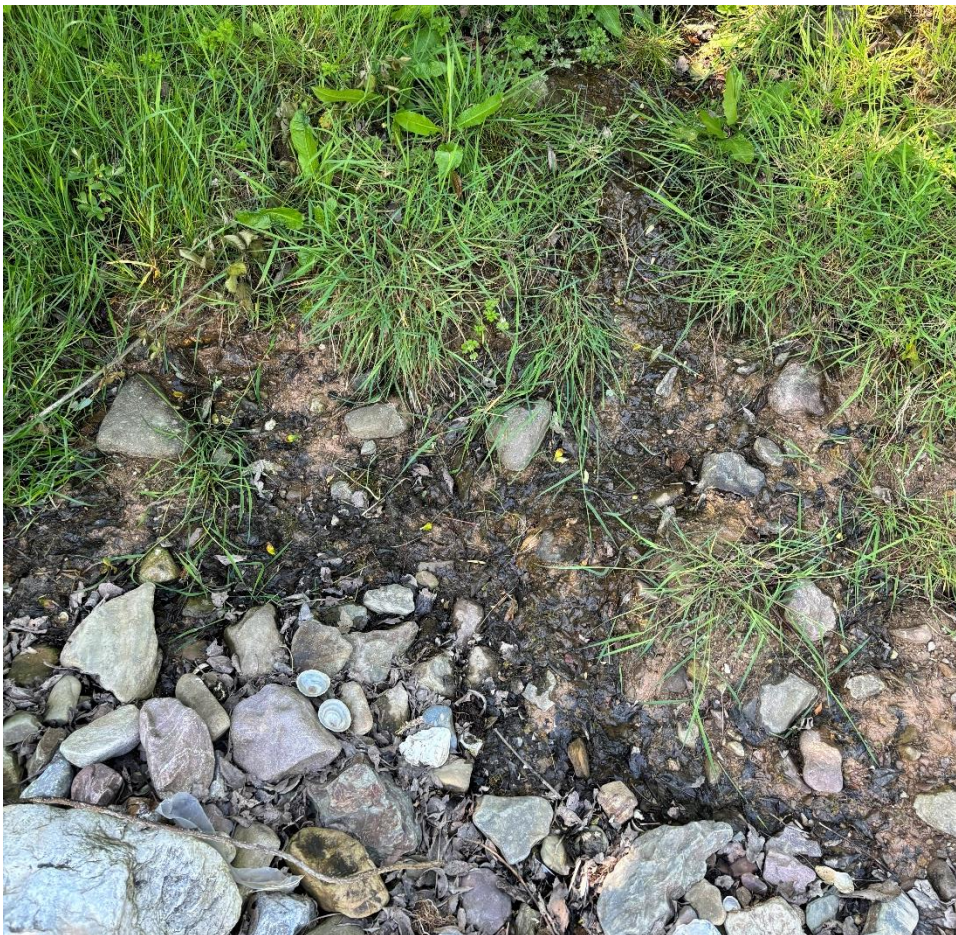
Figure 18 View of the seepage at the cliff toe mid-way between cross-sections E and F
