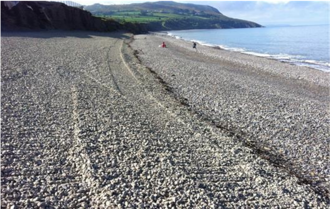
Figure 41 Completed beach nourishment works at Greystones in the area between the revetment and the Gap Bridge. Site visit 25 May 2014
